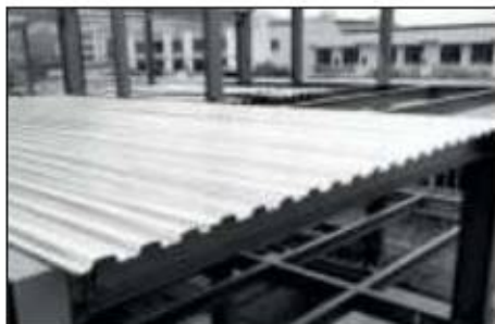
Steel deck and metal roofing
