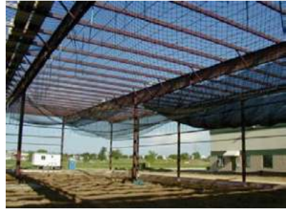
Safety nets used in construction sites.
