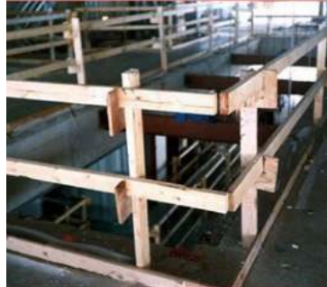
Properly installed guardrail system.
