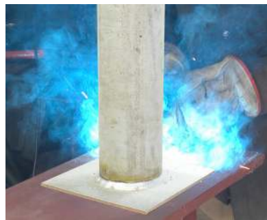
Fig.11 Field Welded Base Plate
