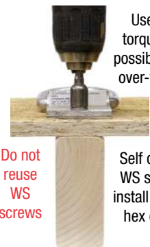
Fig.5 WS Screw Installation
