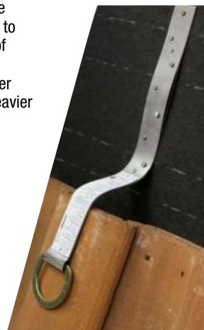
Conform Anchor Leg to the tile profile.
