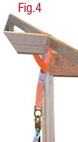
Blocking over Tie-Off Strap will require cutting to evacuate
