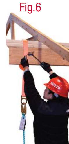
Nail strap to prevent unwanted horizontal movement.
