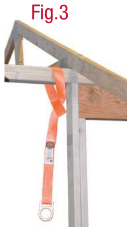
Double top plate required WARNING! Do Not attach to single top plate.
