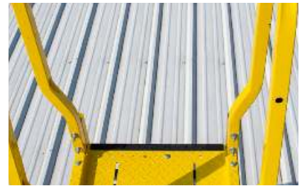
Flat Top Roof Surface
